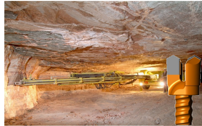
BLAST HOLE DRILLING
